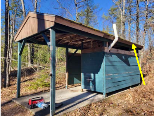
General view of Building, location of roof shingle samples
